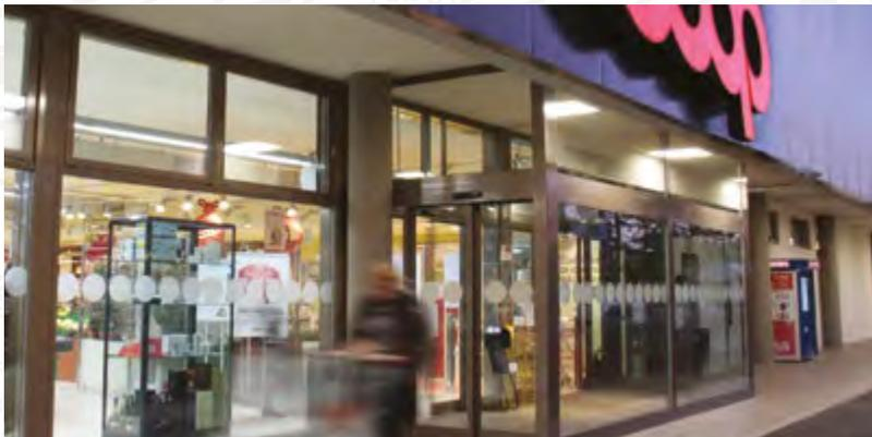
Bussola ingresso a tenuta aria composta / Entrance made of 3 automatic doors for air insulation
